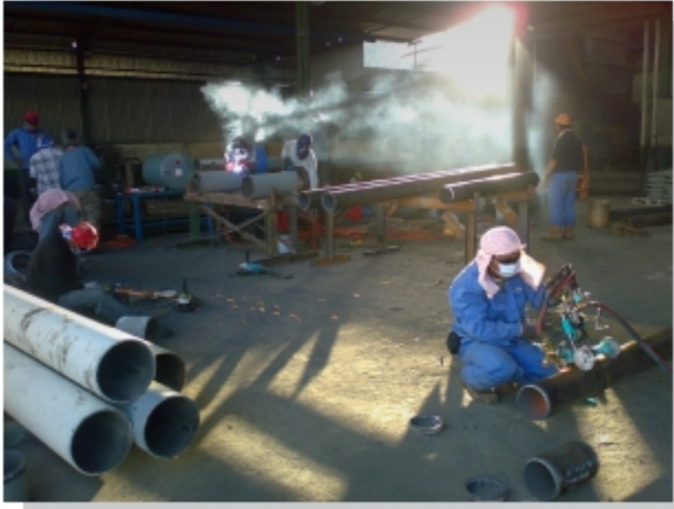
Pipe Shop Welding
