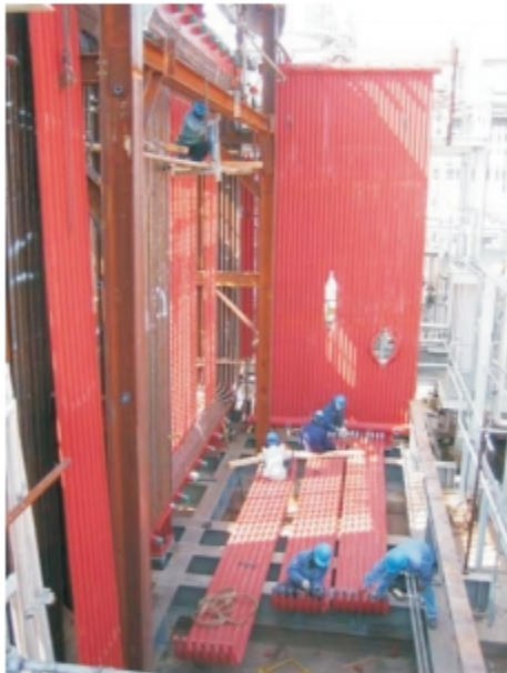
Boiler Tube Installation
