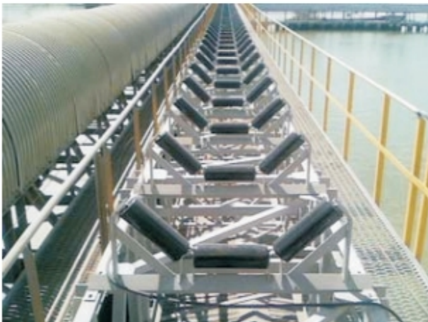
Conveyor Fabrication & Installation
