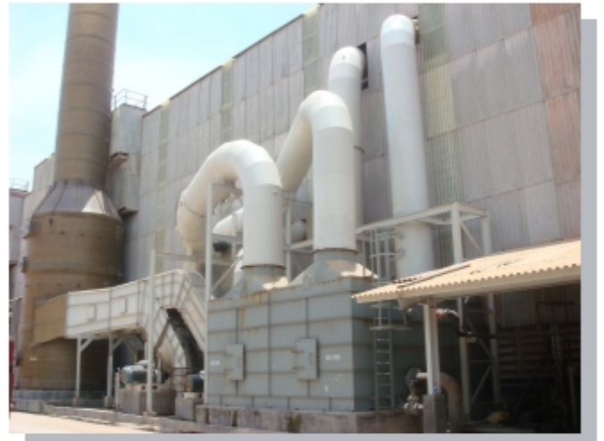
Hot Gas Duct Fabrication & Installation
